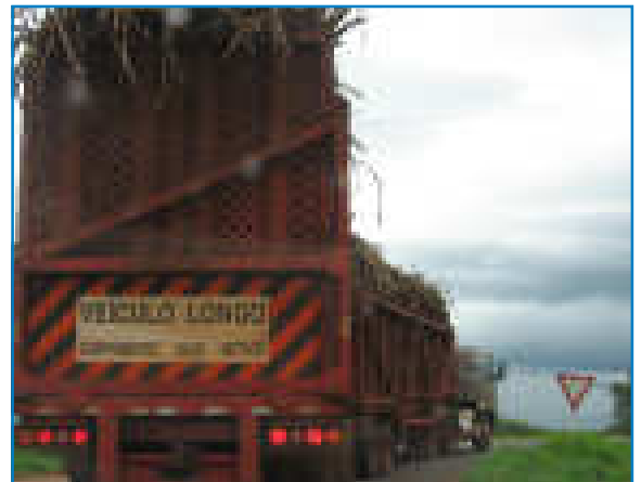
Highway MG 255, Minas Gerais Triangle, December 04, 2006: The excessive weight of trucks loaded with sugar cane has damaged the road surface.
